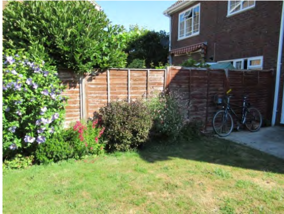
Boundary fence to the right side at the back is worn
