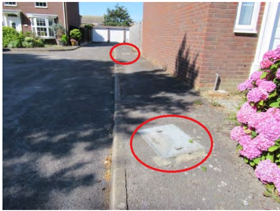
Raised manholes in the footpath to the left side
