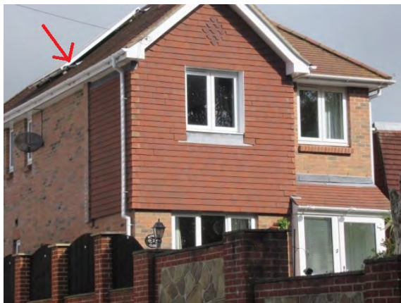
Solar water heating panels on the left side roof pitch
